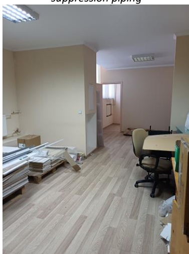
Photo 3. Office space with finished laminate flooring
