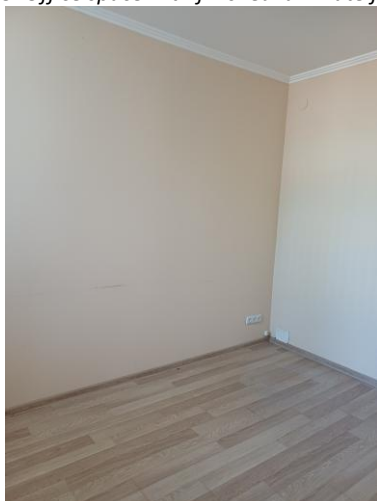
Photo 5. Office room, finished, ready for fit-out
