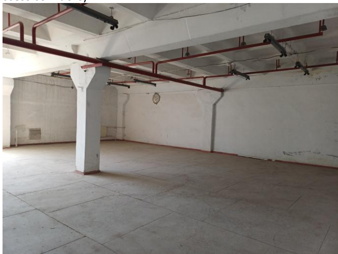
Photo 1. Warehouse / logistics space, with support columns and fire-suppression piping
